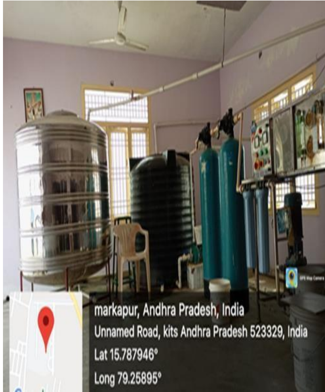
Figure 4 RO water plant providing drinking water
