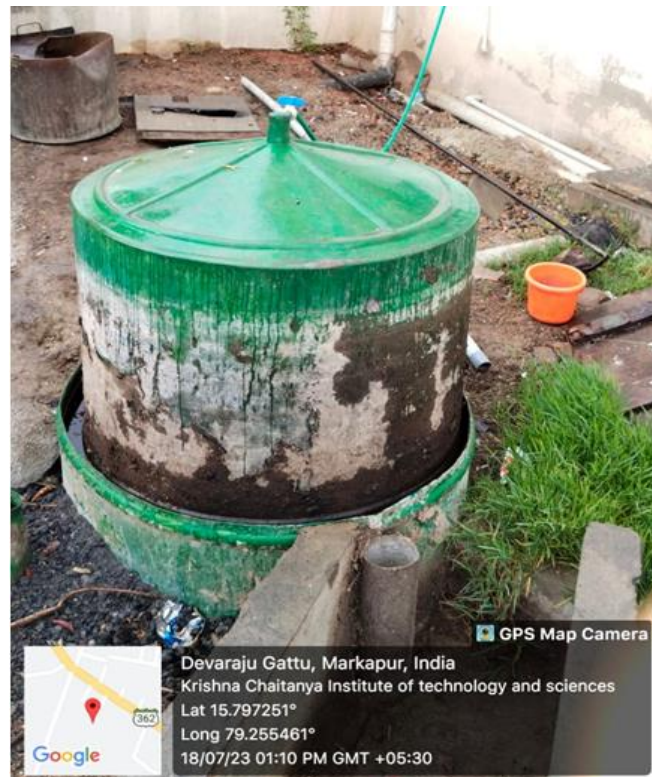
Figure2 Gober gas plant
