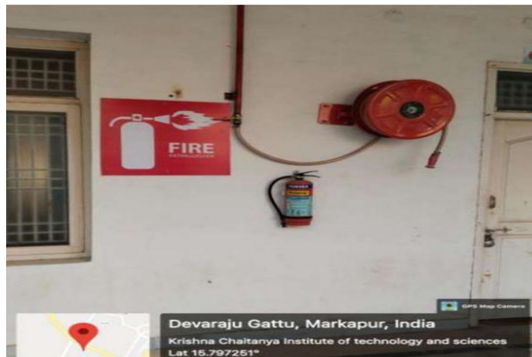
Fig17 : Water distribution utility System in campus
