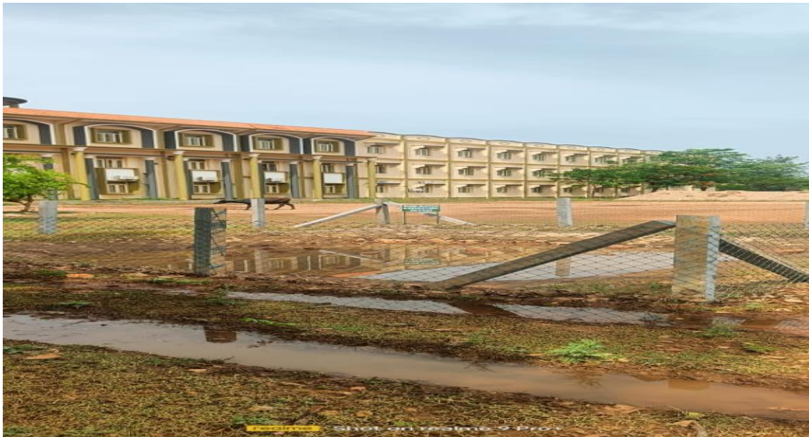
Fig 5 : Rainwater harvesting Ditch-2 at C-Block
