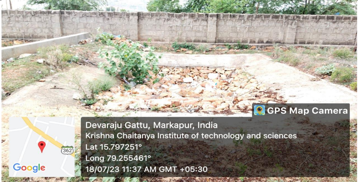
Fig 8: Rainwater harvesting Ditch-5 at A-Block Opposite
