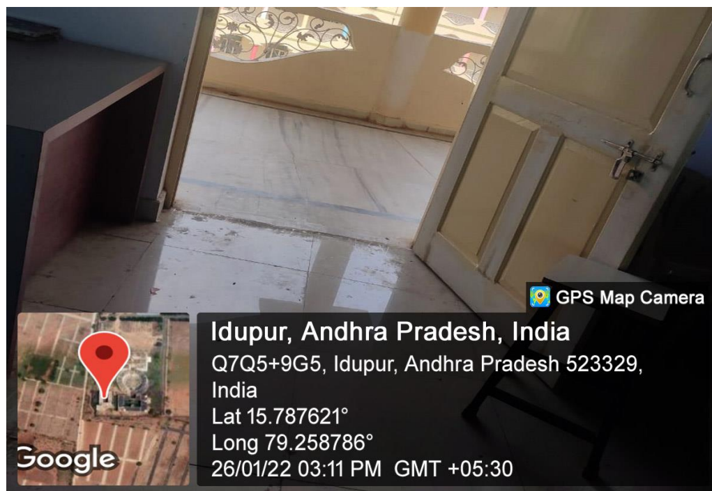
Figure 2 Barrier free class rooms/laboratories
