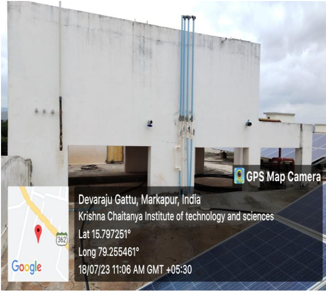
Fig 11 : Overhead Water tank at Block-A
