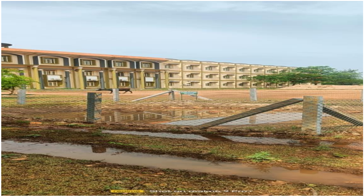
Fig 5 : Rainwater harvesting Ditch-2 at C-Block
