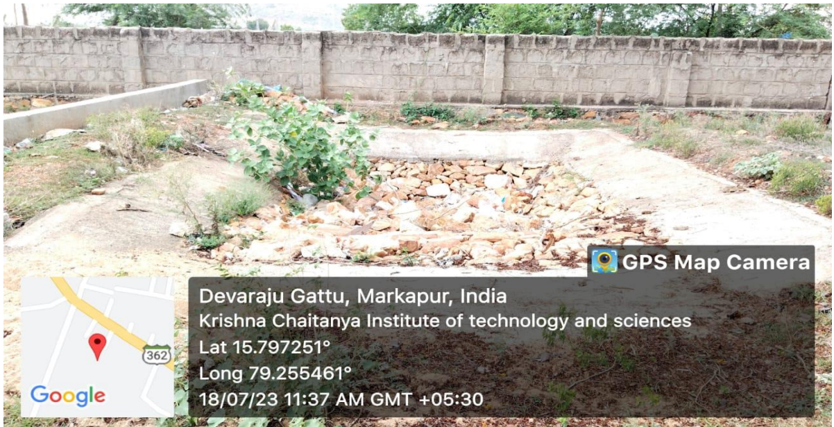
Fig 8: Rainwater harvesting Ditch-5 at A-Block Opposite
