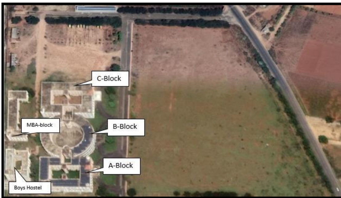
Fig 1: Different building roofs with rain water holding capacity
